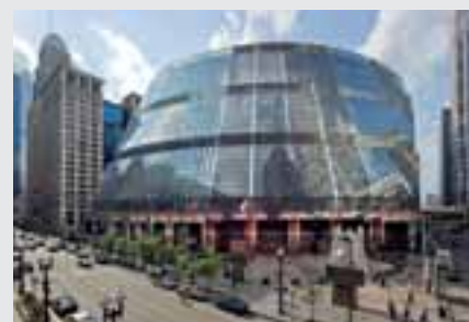
State of Illinois Center, Chicago, 1979–83 Foto: R. Viertlböck © Murphy/Jahn
